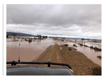
Council's road network and surrounding lands were historically dry at the time of the flood. Consequently, road surfaces and pavements were extremely vulnerable to washing of dry, finer materials from the structure of pavements, floodways, road-related embankments etc. Further, paddocks were "bone dry" as well, vegetation was in poor condition and highly susceptible to being carried away by stormwater washing across paddocks.
