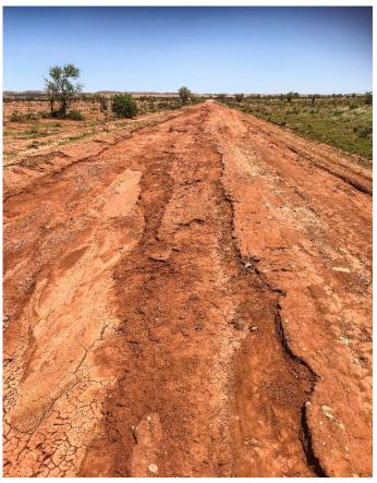
In addition to direct scouring from fast-moving stormwater, large quantities of damaging material and debris were deposited on roads, in culverts (causing blockages and overtopping damage).
