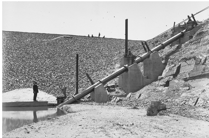
Pekina Creek Dam 1907
