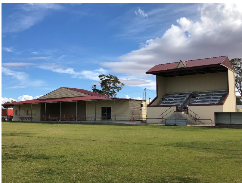
(Stage 1 of the new complex pictured next to the existing Grandstand. Image credit Jodie Bouilly)
