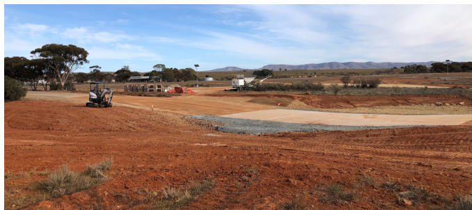
Above: Recent repairs on Wilmington Road
